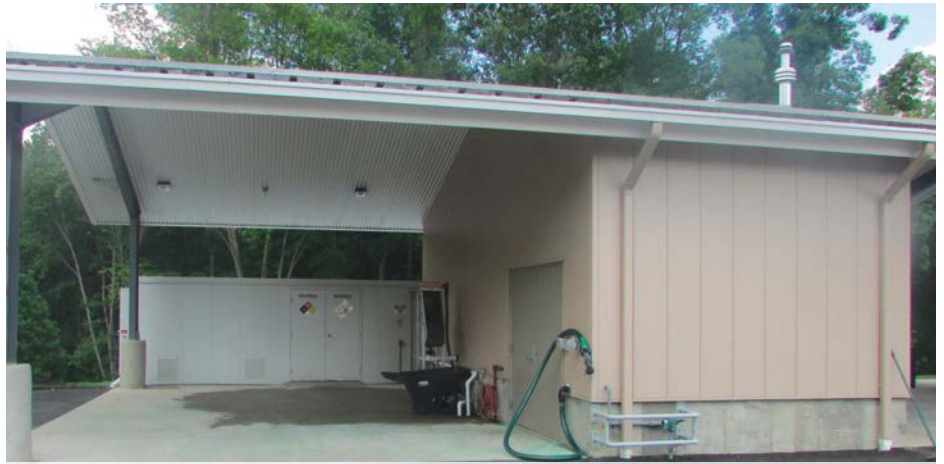
This view of the new maintenance facility at Century CC in Purchase, N.Y., gives no clue of the 6,000-square-foot drive-in basement. Photo by Kevin Seibel, CGCS
